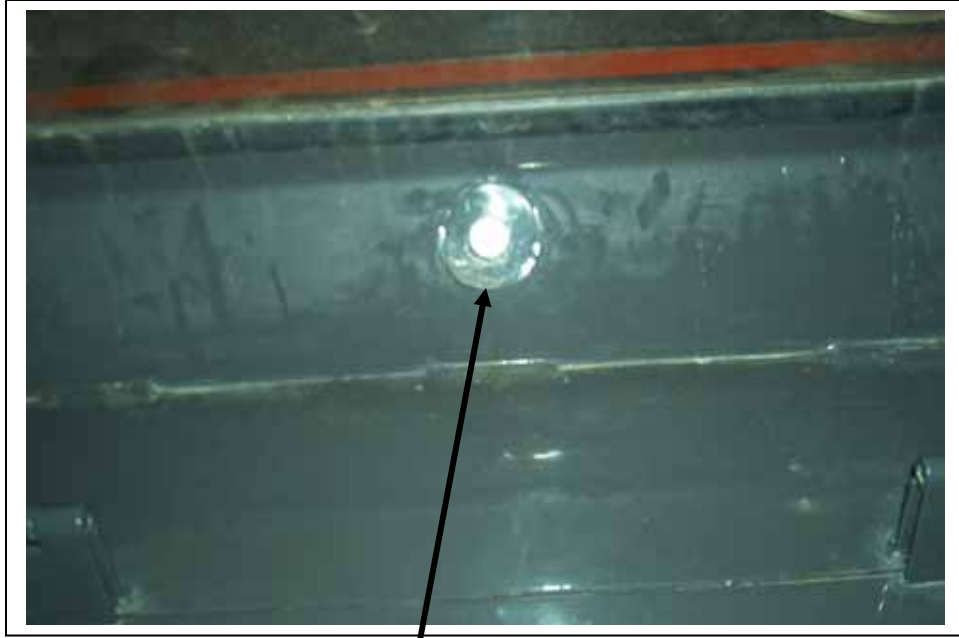
Fifth cab mount bolt at rear window in cab.
