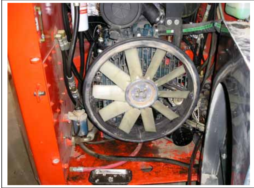
Fan back in place
