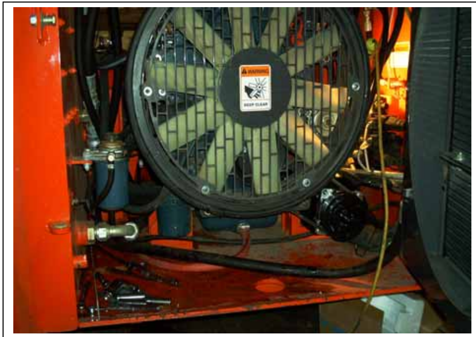
Compressor in place with fan and guard re-assembled.
