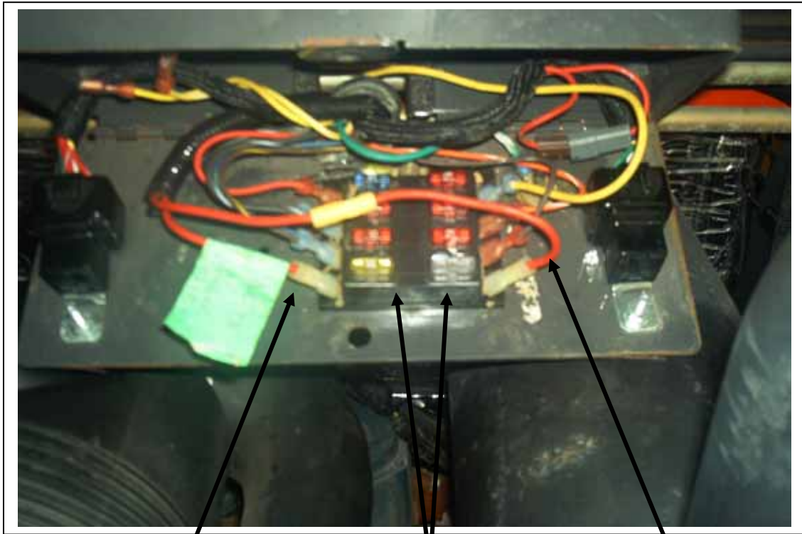
Power wire for relay
