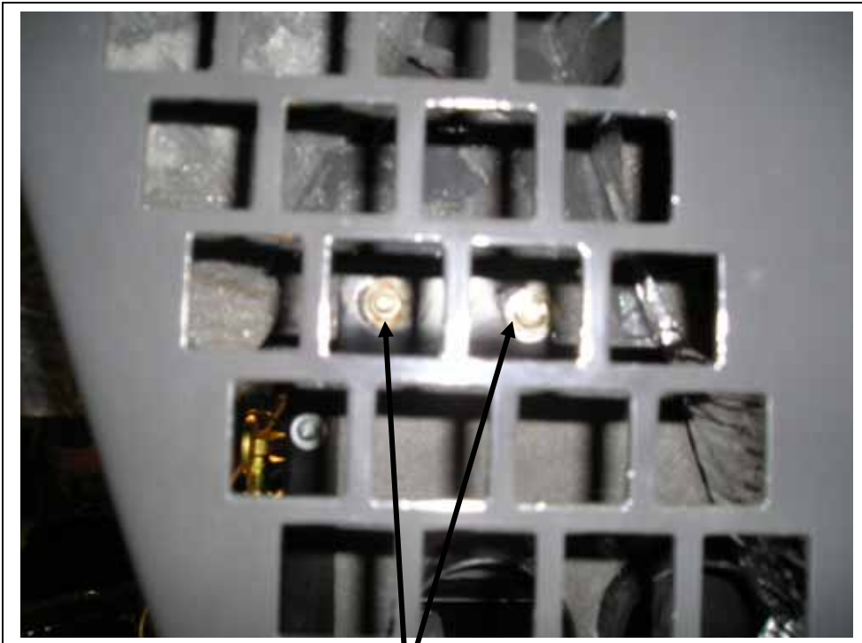
Top two 1/4" mount bolts on the A/C box drilled into the side of the battery box. Use a long 1/4" drill bit to make these holes.
